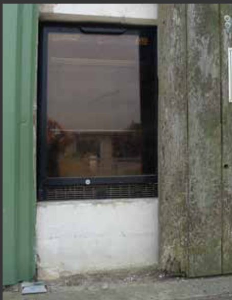
Example for semen drop-off place: Thermocabinet which can be filled from outside the building
